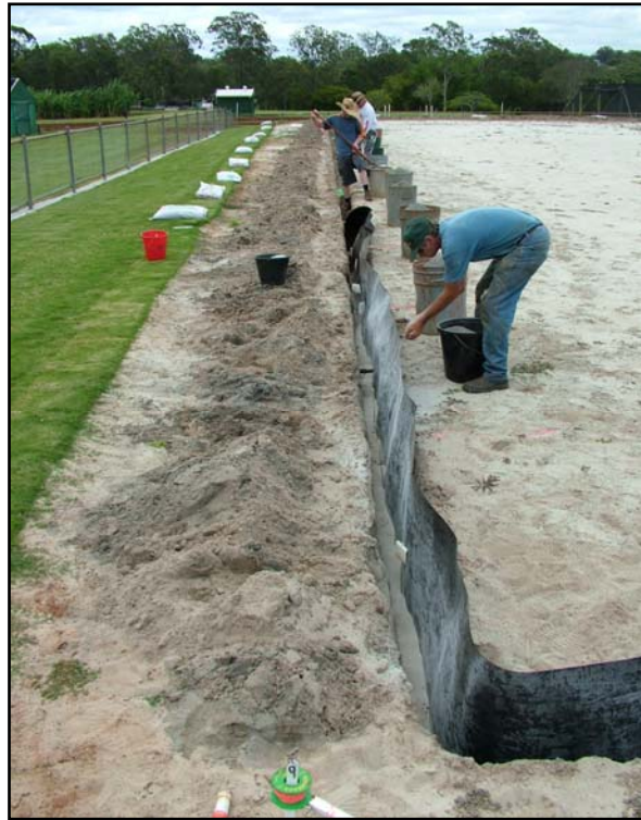
Plate 5. Installation of Root Barrier® and sodium bentonite (sealant) around the perimeter of the DEEDI greens test facility to stop encroachment from green surrounds.
